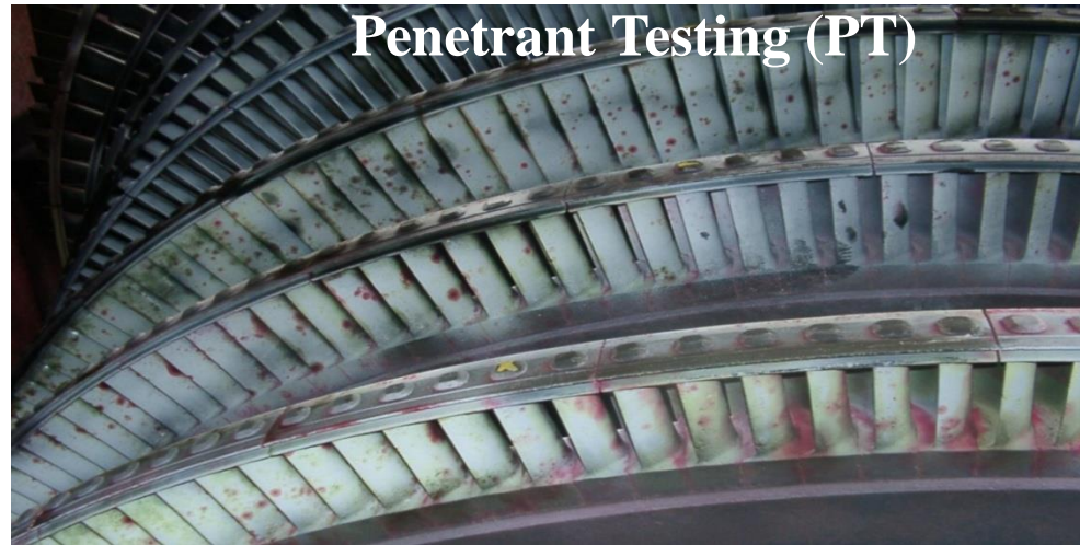
Typical pitting corrosion on 5 th , 6 th and 7 th stage
