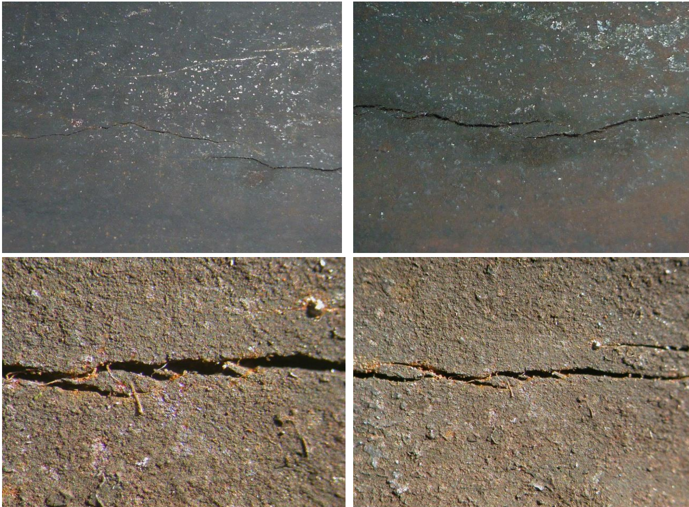
Fire side cracks at the tube internal tube surface
