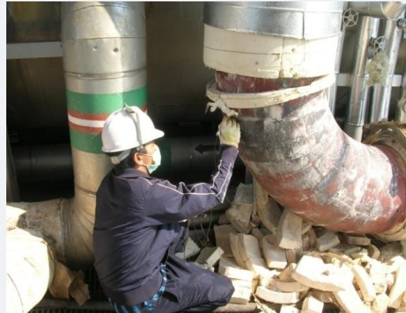
WALL THICKNESS MEASUREMENT
