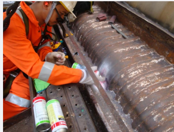
DYE-PENETRANT TEST (PT)
