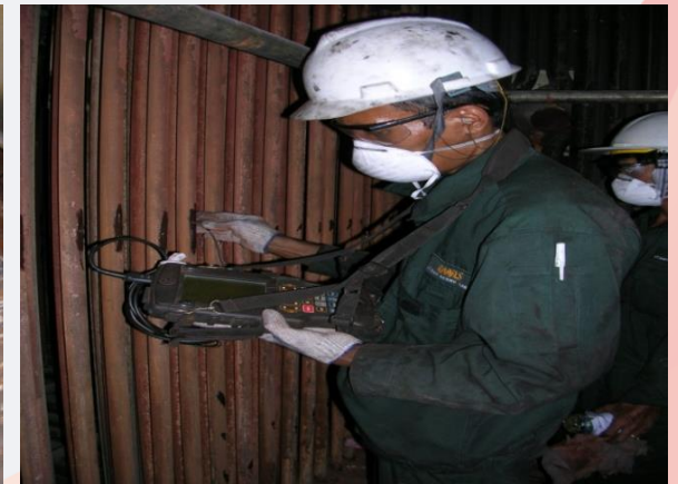
WALL THICKNESS MEASUREMENT
