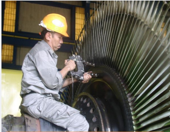
MAGNETIC PARTICLE TESTING (MT)
